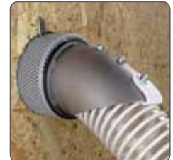
4 The corners of the stud cavity can also be filled by rotating the nozzles head.
