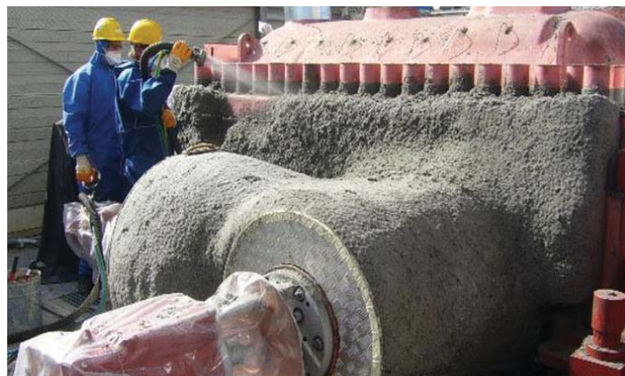
Application : Isolation technique
