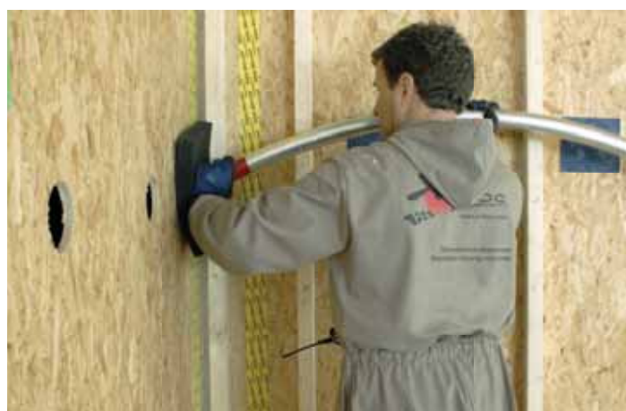
Injection needles are also ideally suited for filling hard-boarded compartments
