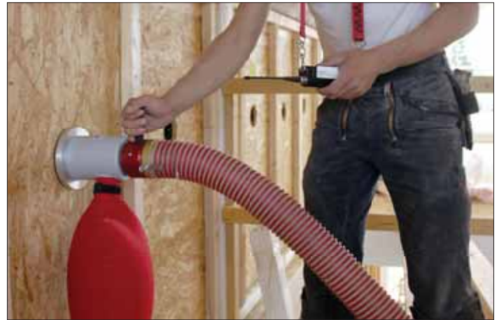
Dry injection with a ventilated rotary nozzle
