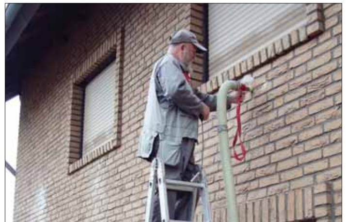
Cavity wall insulation
