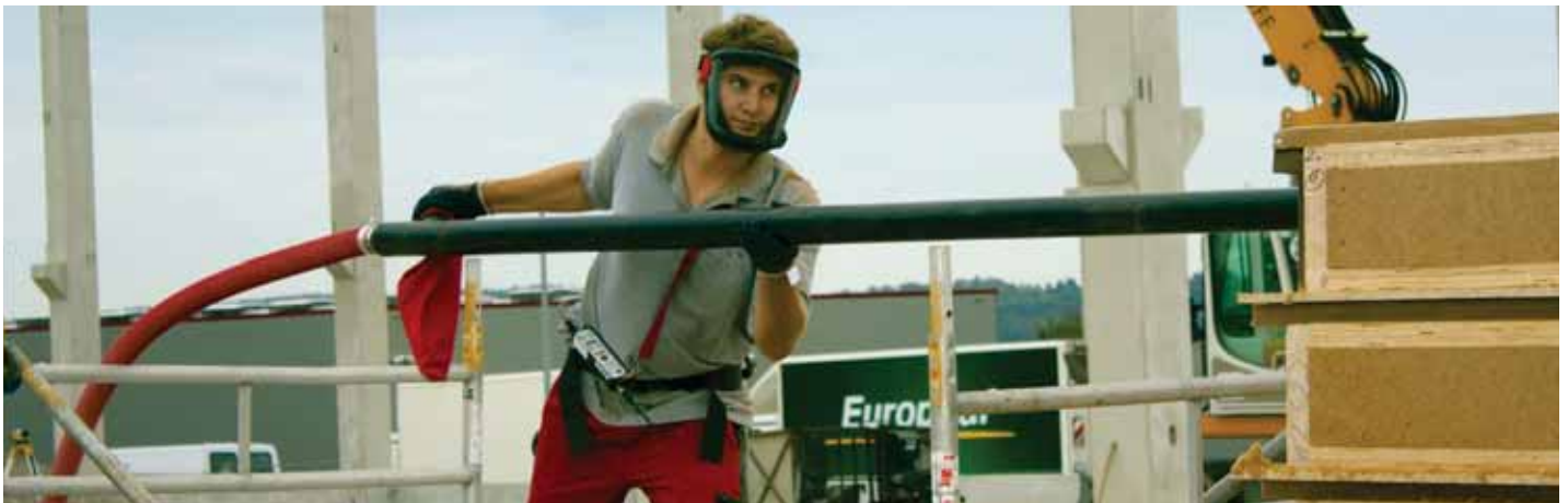
Industrial-grade element filling with the aid of vented injection lances
