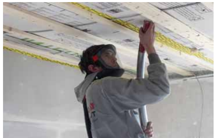
Injection needle with specially shaped, colour-marked tube tip as a piercing aid
