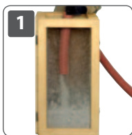
Dry injection with hose
