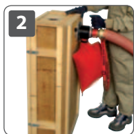
Dry injection with ventilated rotary nozzle
