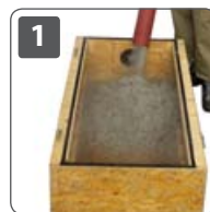
Open blowing with hose
