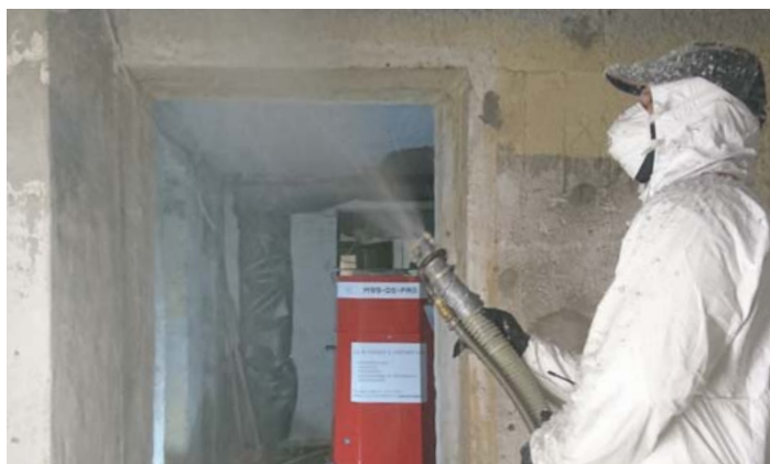
Frequently used for damp spraying: the mobile all-rounder X-Floc Minifant M99
