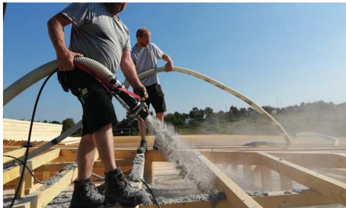
...in use for power damp spraying
