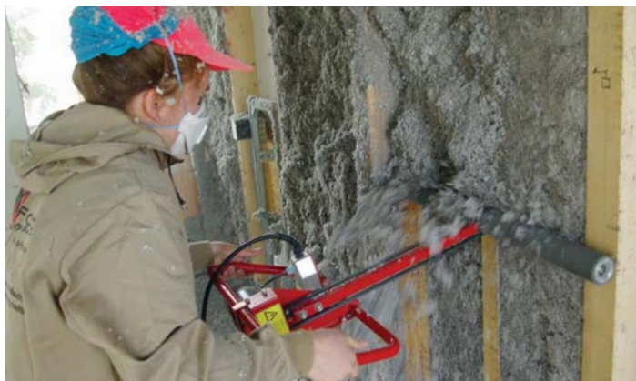
Surface smoothing with the wall scrubber M05
