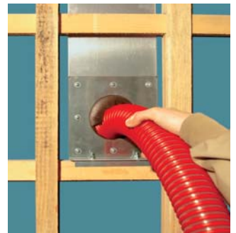
Insertion of the injection hose
