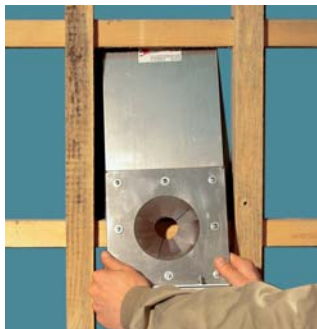
Placement between the battens
