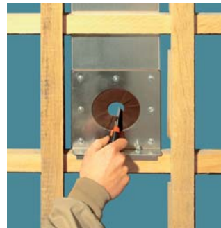
Manufacture of blowing hole
